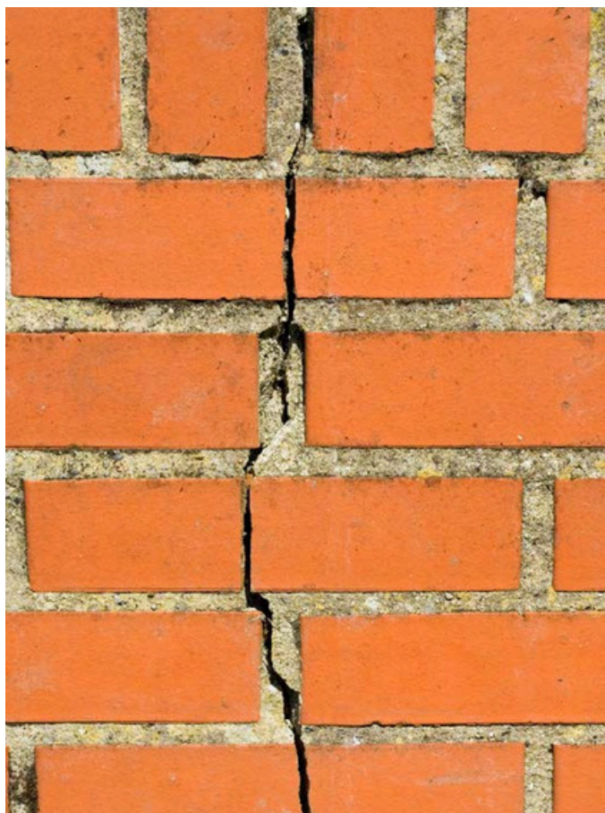
Wall Cracks
