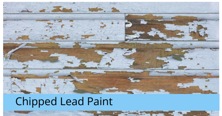
Chipped Lead Paint
