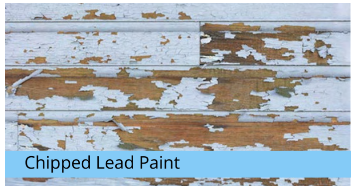
Chipped Lead Paint
