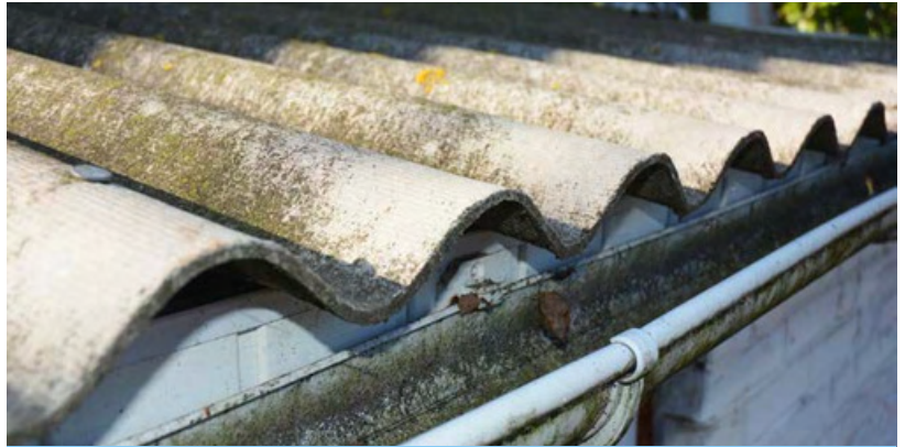
Asbestos in Roofing Materials
