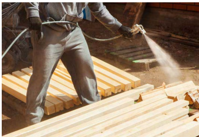
Spraying of Flame Retardant on Dressed Lumber
