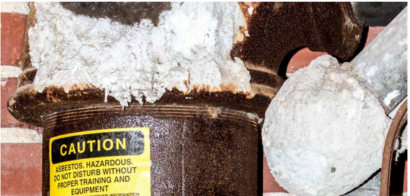
Asbestos on Pipes
