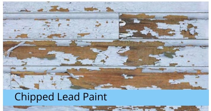
Chipped Lead Paint
