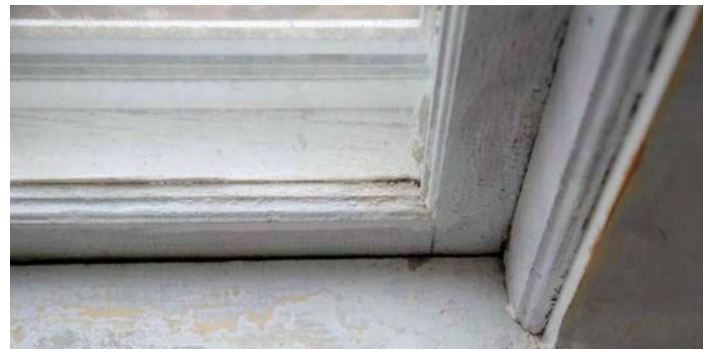
Chipped Lead Paint
